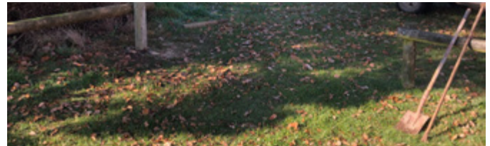
Entrance near the Rec Centre repaired.
